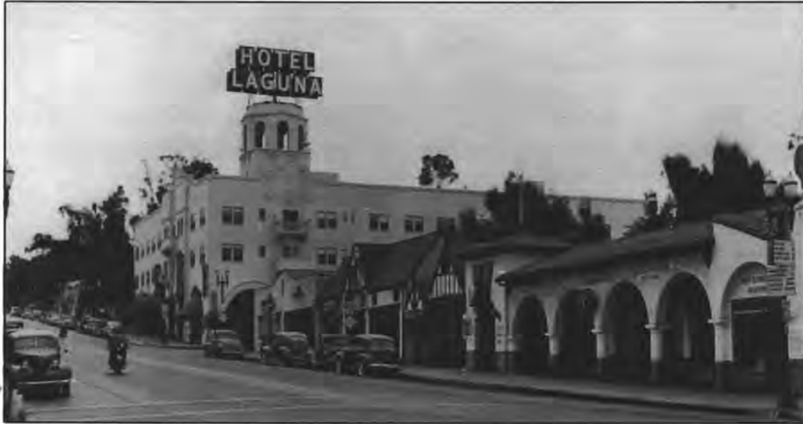
1940's Hotel Laguna with neon sign on top. The sign, which was removed in the 1960's, was considered a Landmark. In the foreground, the Isch Building, a Mediterranean Revival built in 1927.
