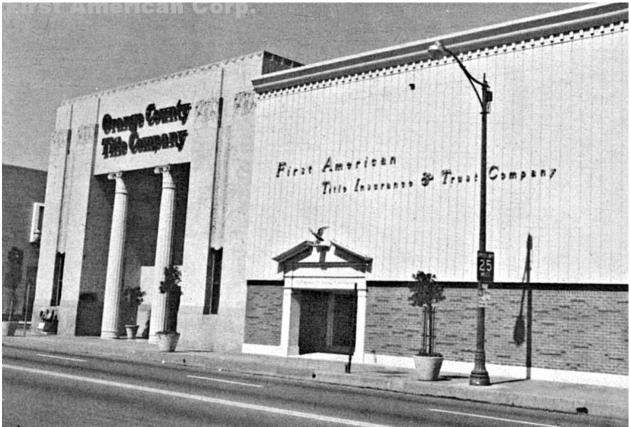
View of First American Title Building, Main Street elevation looking north. photo ca 1963
