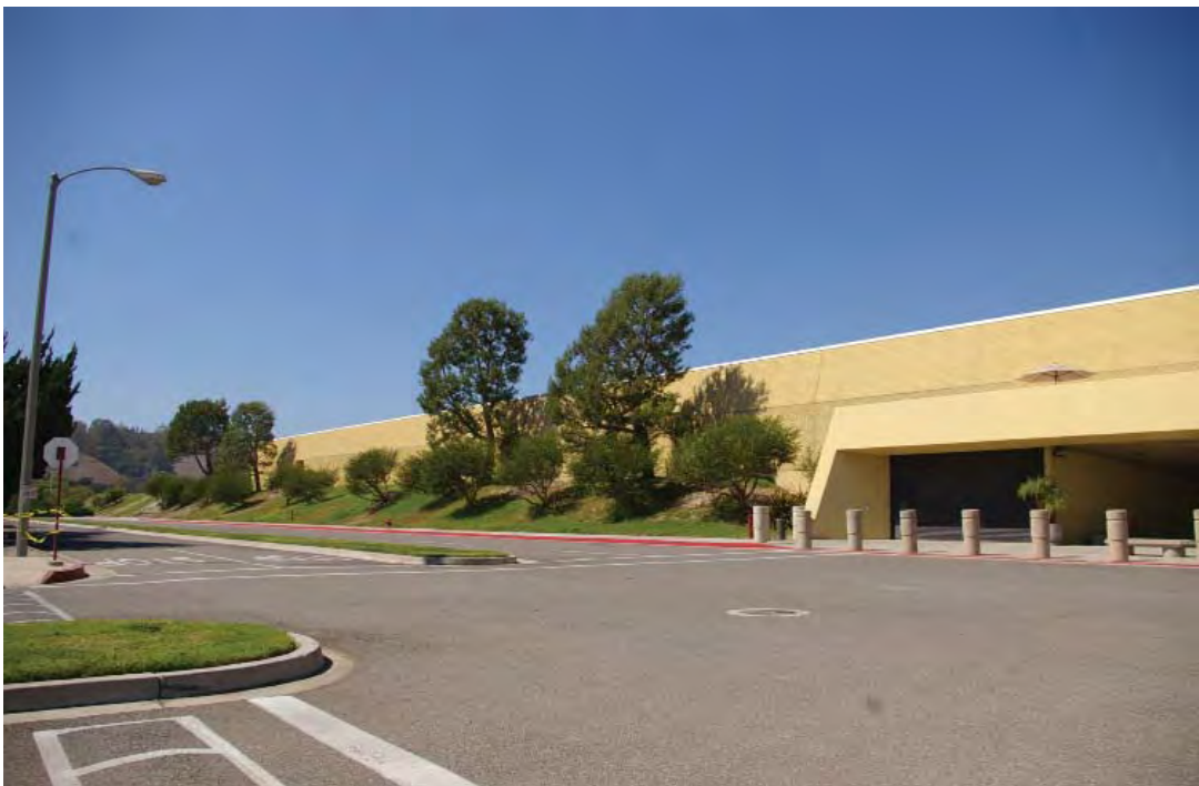
Image 15: The south facade looking northwest toward the south entrance. This entrance now serves as the main public entrance to the building.
