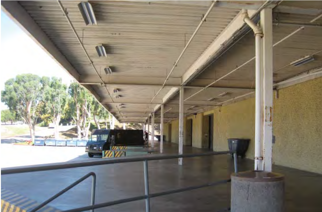
Image 18: The loading dock on the west facade of the building.
