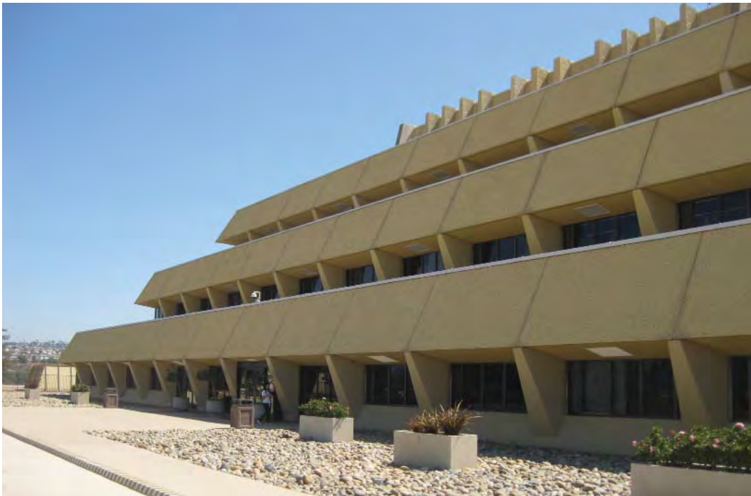
Image 9: The original main entrance located on the north facade.
