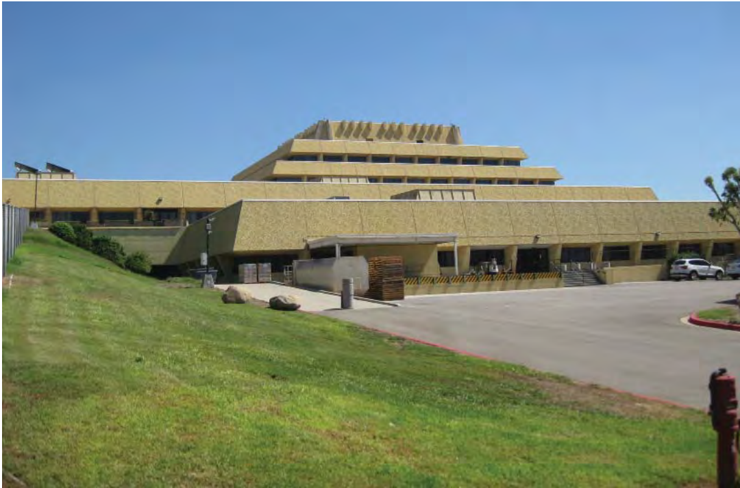
Image 16: The west facade looking southeast toward the loading dock.
