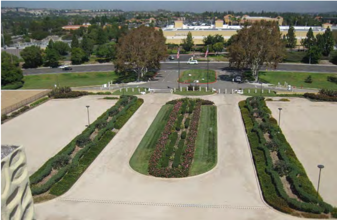
Image 10: The parking area at the north side of the building looking down from the roof.
