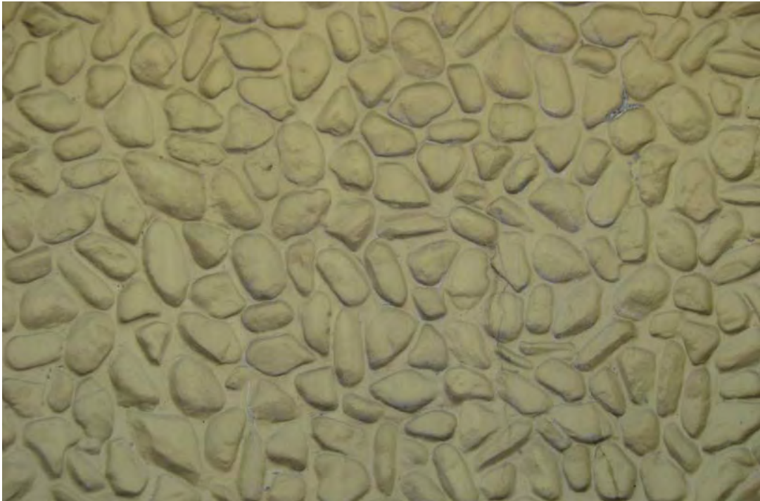
Image 22: Close-up view of the typical exterior wall finish. The pre-cast concrete panels have a pebble texture.
