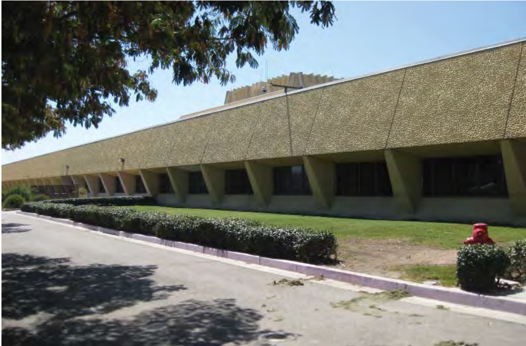
Image 12: The east facade looking southeast.
