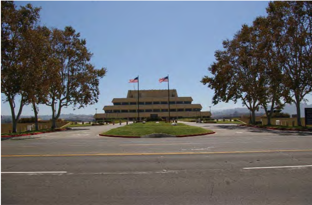
Image 8: The original main entry to the Chet Holifield Federal Building on the north side of the building. The entry drive leads to two parking areas which are located on top of the third floor roof deck. These lots are currently closed and the main public entrance has been moved to the opposite side of the building.
