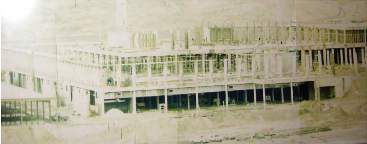
Image 2: The Chet Holifield Federal Building under construction. (Source: General Services Administration.)
