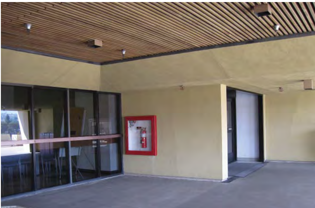
Image 29: A covered vestibule at the outdoor dining area. The wood ceiling finish is original. The same detail is used at other primary interior spaces including elevator lobbies, escalator areas, and the south entrance.
