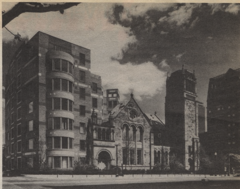
Graham Gund Associates of Massachusetts fashioned Church Court Condominiums around the ruins of a 19th-century Boston church.
