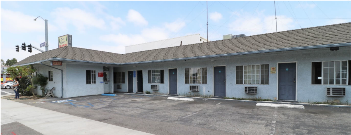
Figure 15: South elevation of the motel, view to the northwest (6/4/2020).
