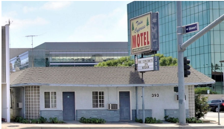
West elevation of the Twin Cypress Motel, view to the east (6/4/2020). Note missing door where street numbers are and the relocated pole sign.
