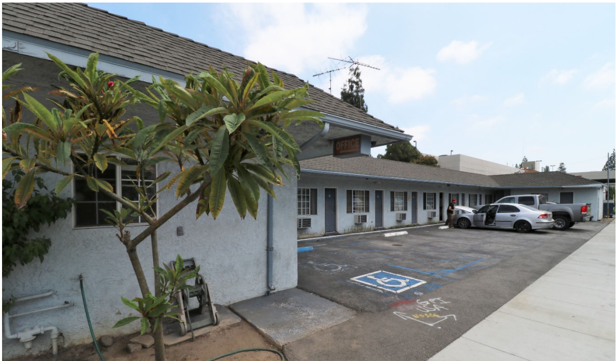
Figure 14: South elevation of the motel, view to the northeast (6/4/2020).
