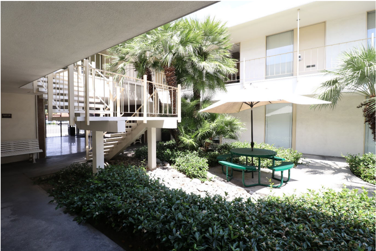
Figure 9: Atrium. View to the northwest (/6/4/2020).
