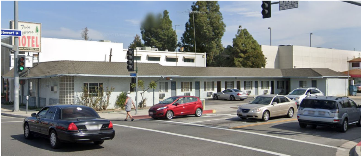
Figure 13: West and south elevations of the Twin Cypress Motel, view to the northeast (Google February 2020). Note two modern windows east of the glass blocks where the postcard showed three.
