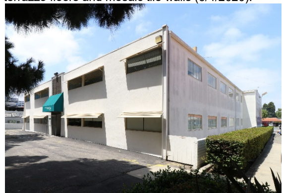
East and north elevations, view to the southwest (6/4/2020).
