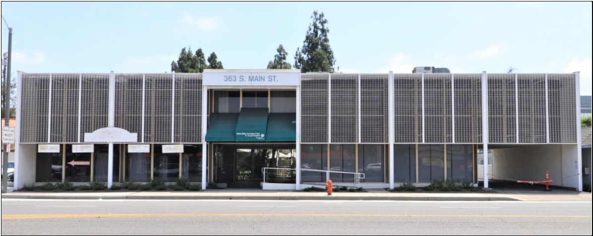
Figure 6: Façade, view to the east (6/4/2020).
