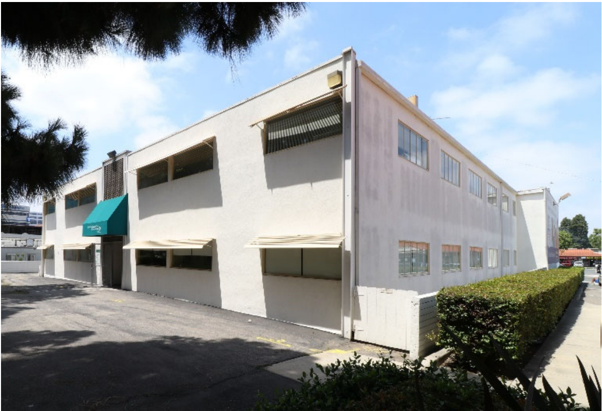
Figure 11: East and north elevations. View to the southwest (6/4/2020).
