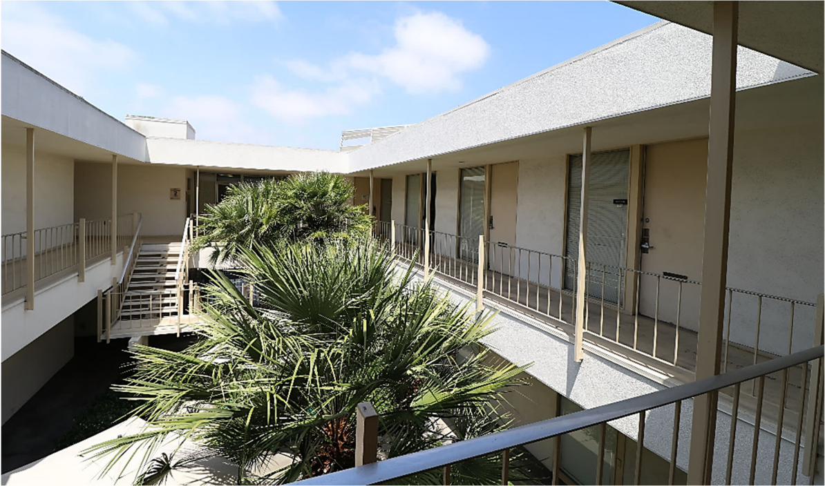
Figure 10: Atrium, balcony, and second floor offices. View to the west (6/4/2020).
