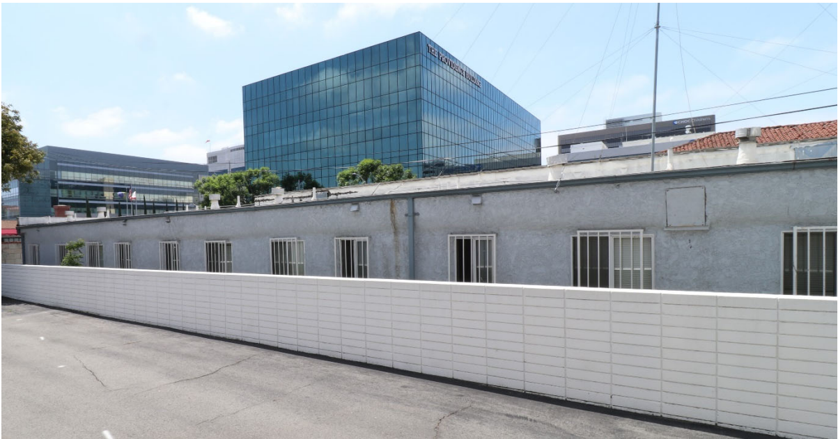
Figure 16: North elevation of the motel, view to the southeast (6/4/2020).
