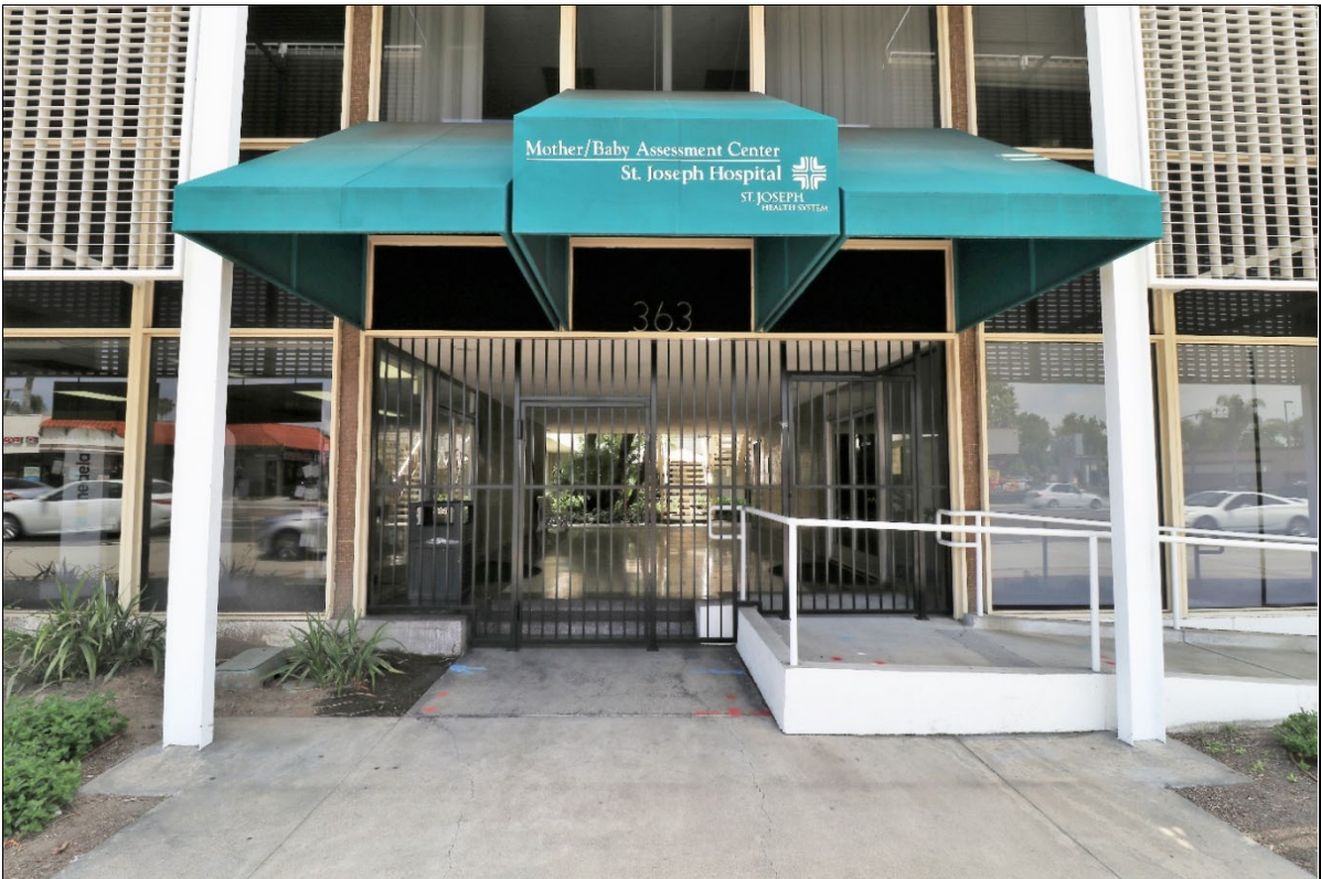
Figure 7: Main entrance. Note alterations: ADA ramp, green awnings, and security bars. View to the east (6/4/2020).
