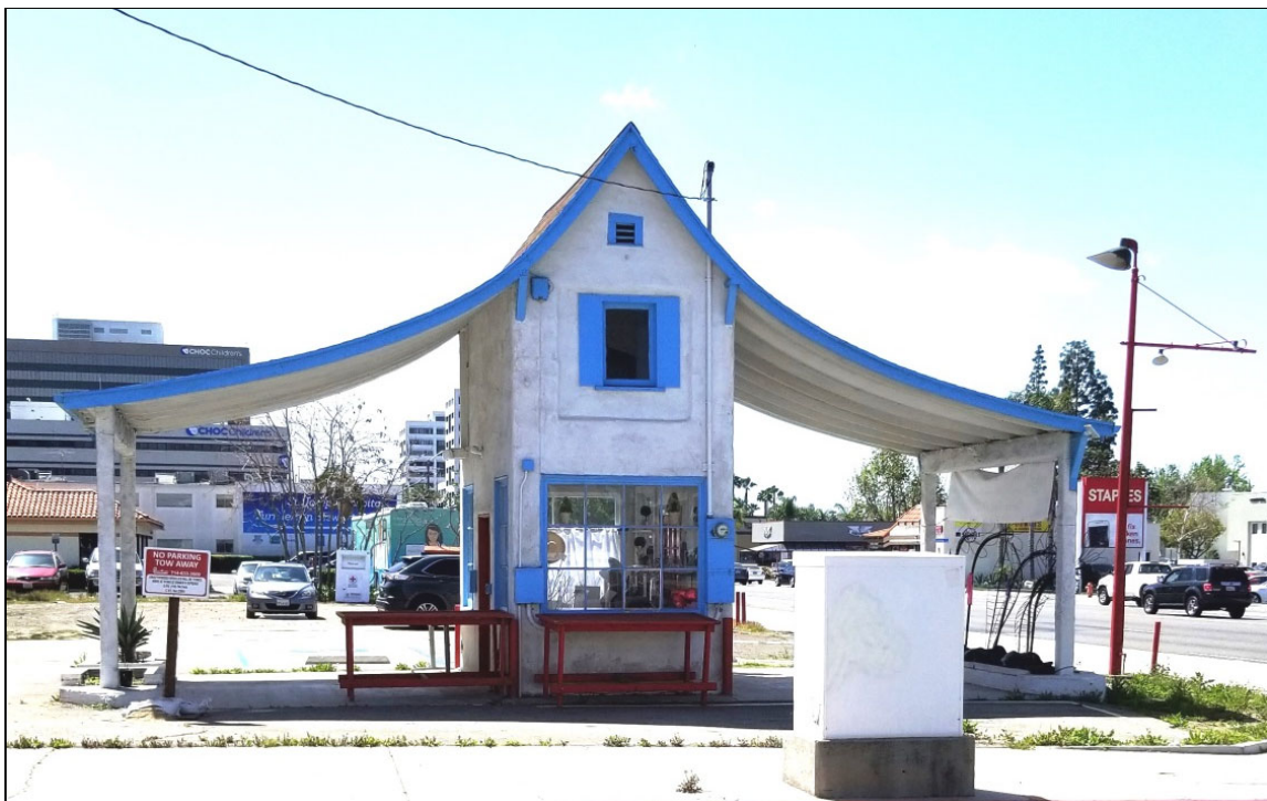
Figure 12: Former gas station, north elevation, view to the south (4/12/18).
