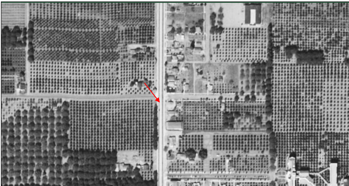
Figure 4: 1931 Aerial Photograph Showing 305 S. Main Street Property. The major north-south street is S. Main Street. Orange County Archives (2020).
