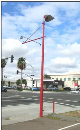
Light standard/mast-arm sign on South Main Street, view to the northwest (10/31/17).
