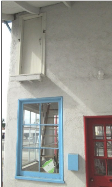
Figure 13: Second-floor door in east elevation (10/31/17)
