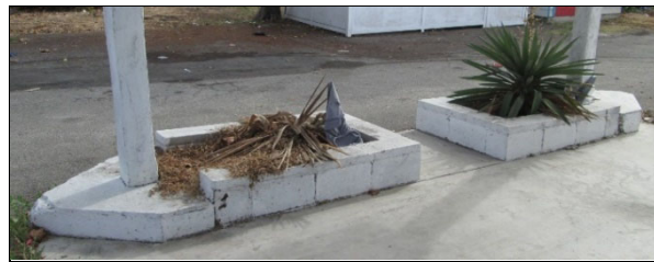
Figure 16: East pump island, view to the east (10/17/31).
