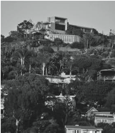
Residential Architecture Halliburton House – Hillside Housing South Laguna Photography – Ann Christoph
