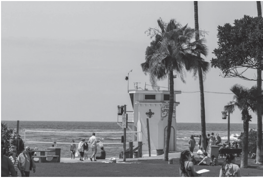
Commercial Architecture Life Guard Tower Main Beach - Pacific Coast Highway Photography – Tom Lamb
