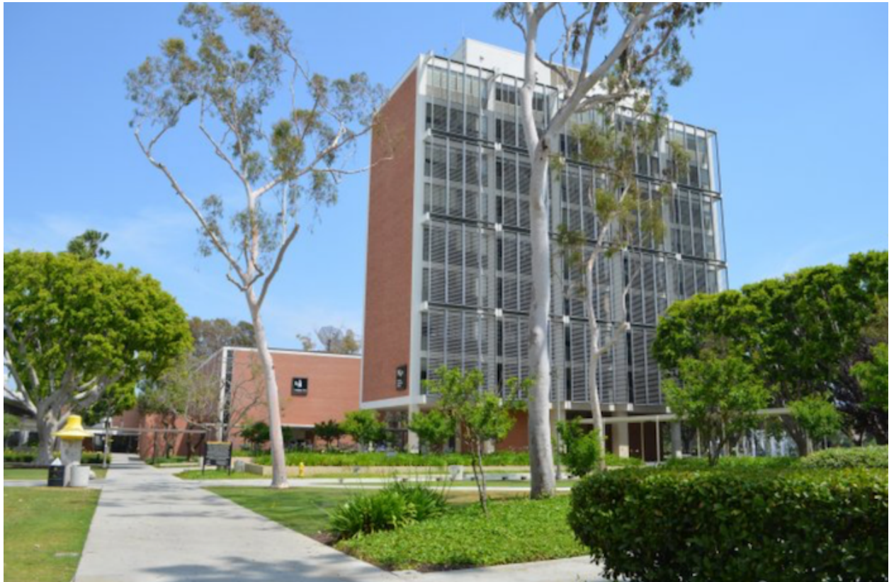
Figure 1.0 McIntosh Humanities Building, California State University Long Beach, CA, 1965 by State Office of Architecture and Construction. Note the metal screen attached to the building's main elevation. Photograph by Sarah Locke/LA Conservancy
